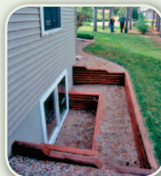
A 3-to-5-foot “fuel free zone” keeps flames away from siding.
